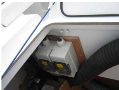
Bipolar circuit breaker (Ref 2)
